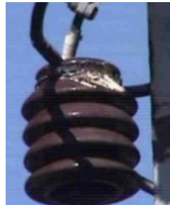
Fig. 9, 10. Corona discharge and its effects.
